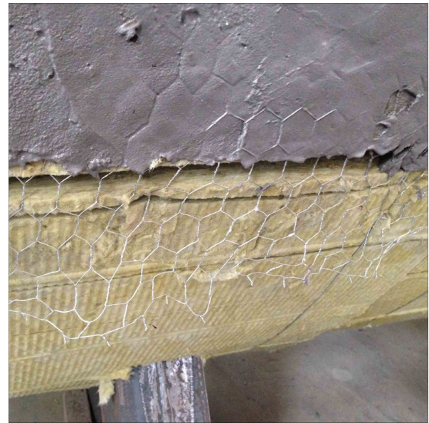
ZOZEN Boilers' Insulation Material 2. (Refractory cement on the rock wool)
