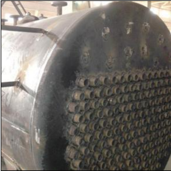
Welding effect from some other boiler factories.
